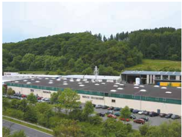
Partial view of the Technitube pipe mill
