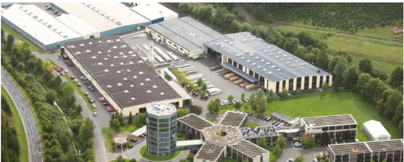
TPS tube mills and bending facilities
